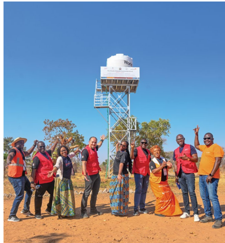
World Vision supports the installation of mechanized water systems that provide safe, clean water to communities like this one in Zambia.
